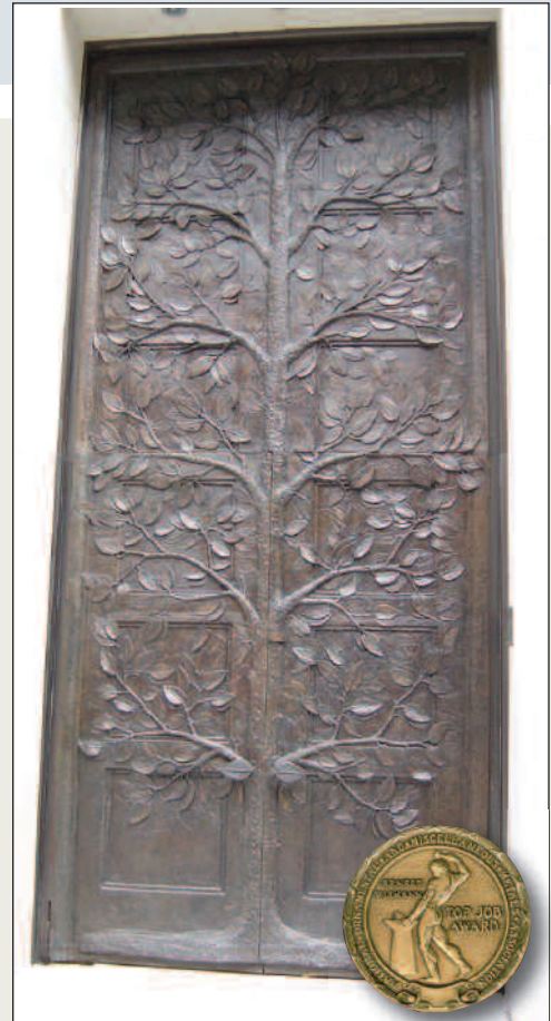
TOP: The ornaments on the front side shell were cast using a loose wax bronze casting and finished to a dark brown patina. The design, which depicts the Jewish Tree of Life, was done by the well-known French architect Thierry Despont. Getting the casted sections to look like a single piece was a challenging part of the job.
